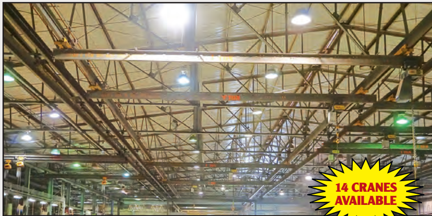
VIEW OF OVERHEAD BRIDGE CRANES
