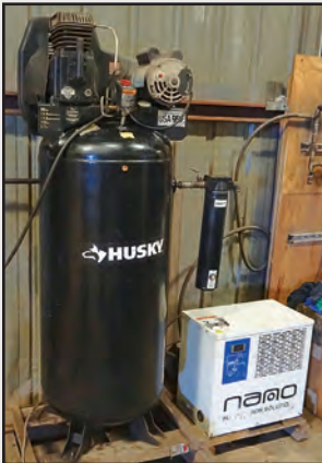
HUSKY AIR COMPRESSOR WITH NANO AIR DRYER
